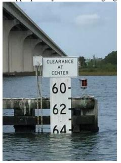
Figure 21. Photograph of a vertical gauge board in service marking how much vertical clearance there is at a bridge.
